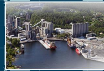
Norcem AS, Brevik Cement plant
